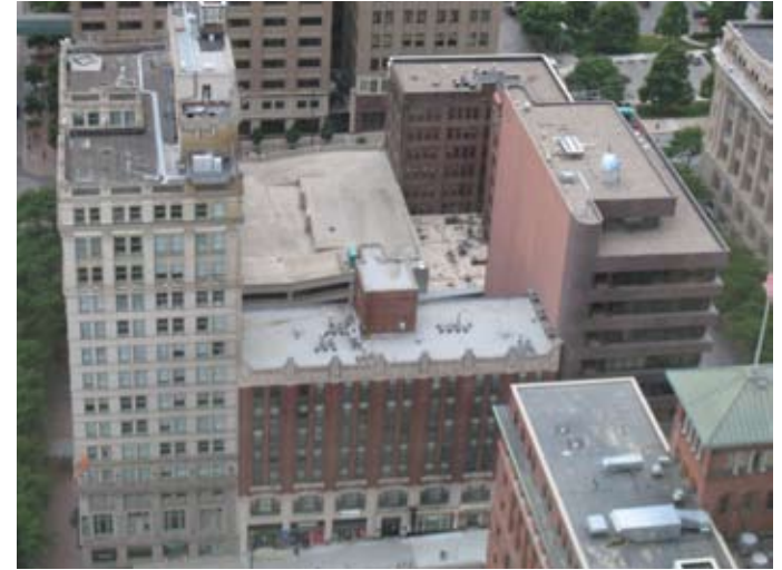
Parking garage built behind historic structures
