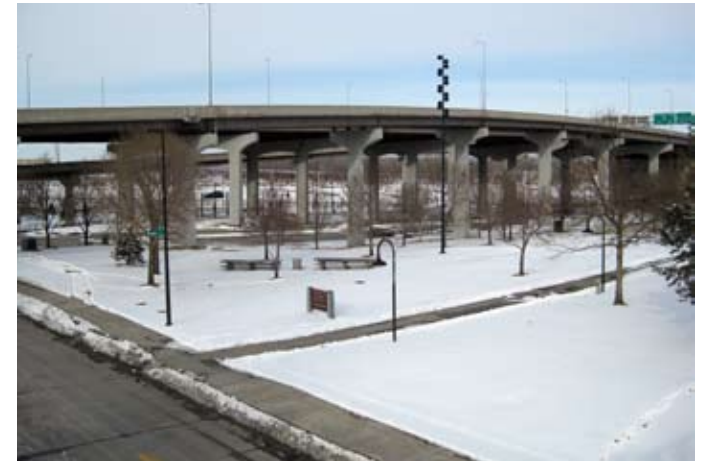
The T-intersection of Douglas Street at 8th Street would connect to an extended Riverfront Drive.
