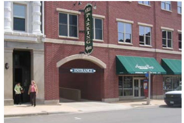
Parking garage tucked behind retail in Dubuque, IA
