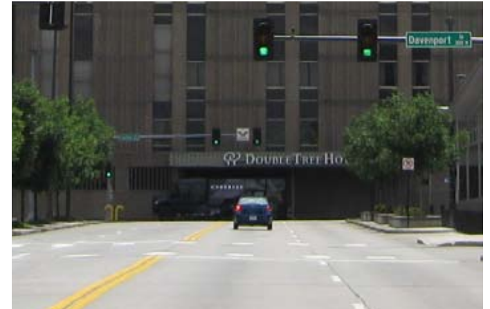
The Double Tree Hotel currently terminates 16th Street
