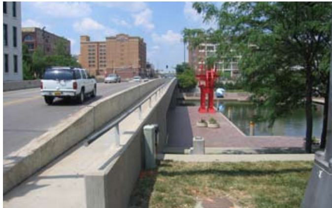
10th Street Bridge looking north over the Gene Leahy Mall
