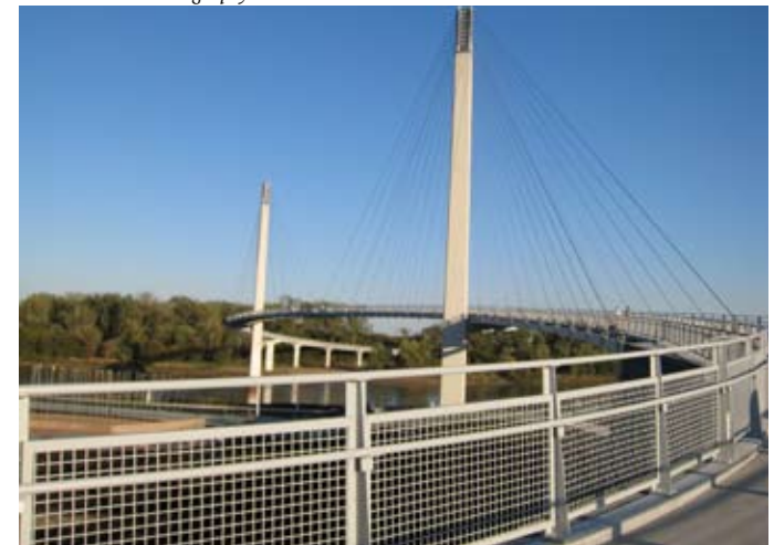
The Bob Kerrey Pedestrian Bridge over the Missouri River
