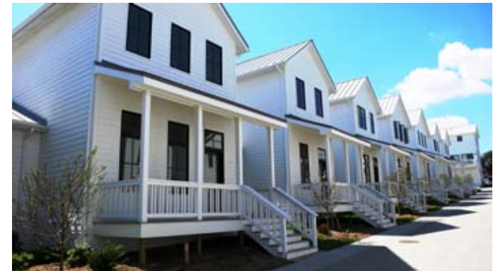
Towns at Little Italy in the Near South District
